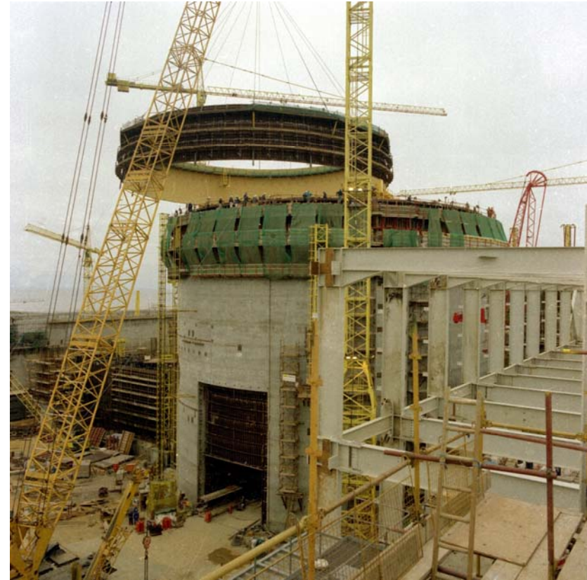
Construction of Sizewell B
