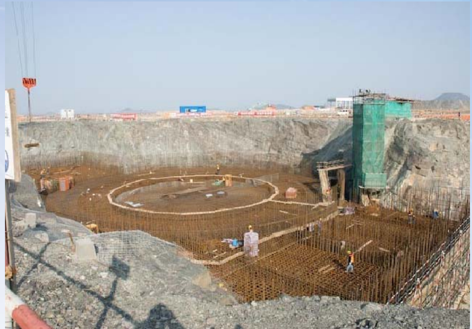
Sanmen Basemat Rebar
