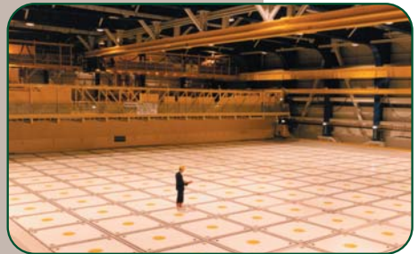
ILW interim surface store
