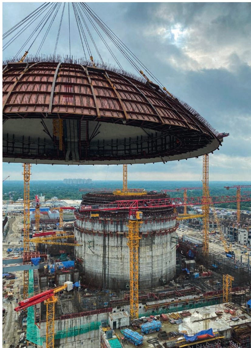
Rooppur under construction (Image: Trest RosSEM)
