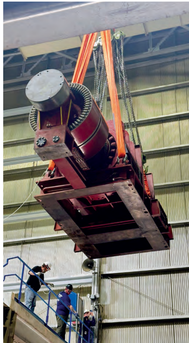
Lifting the Exciter (Image: Holtec)
